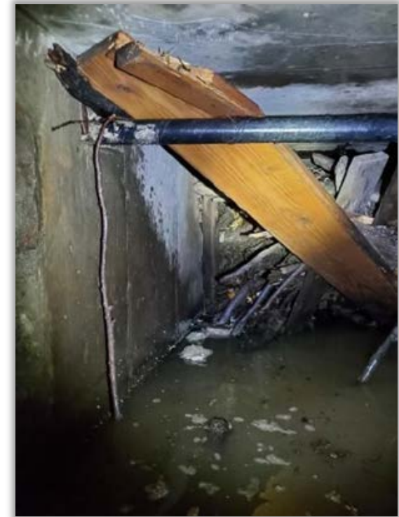
Sediment and debris was removed from stormwater RCB in 2022
